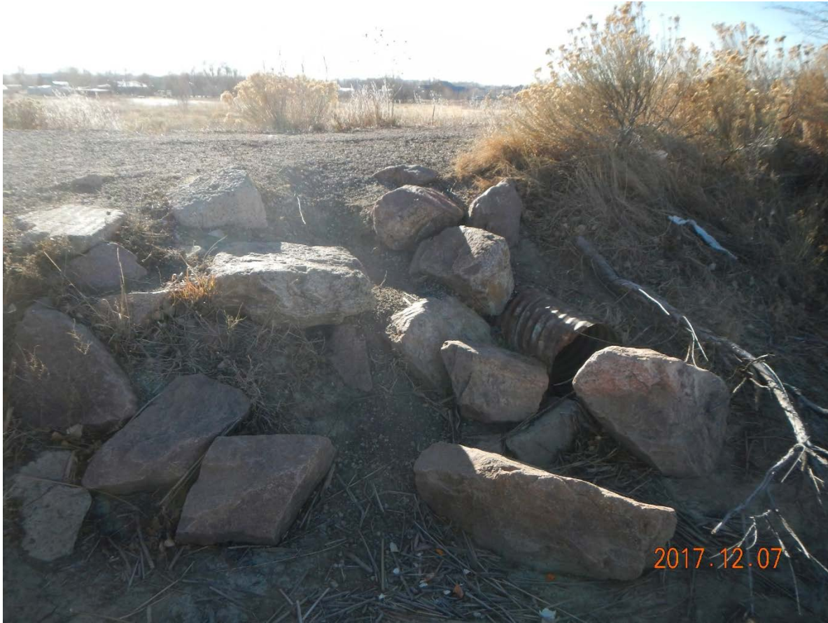
21_Pipe Spillway on left end of dam
