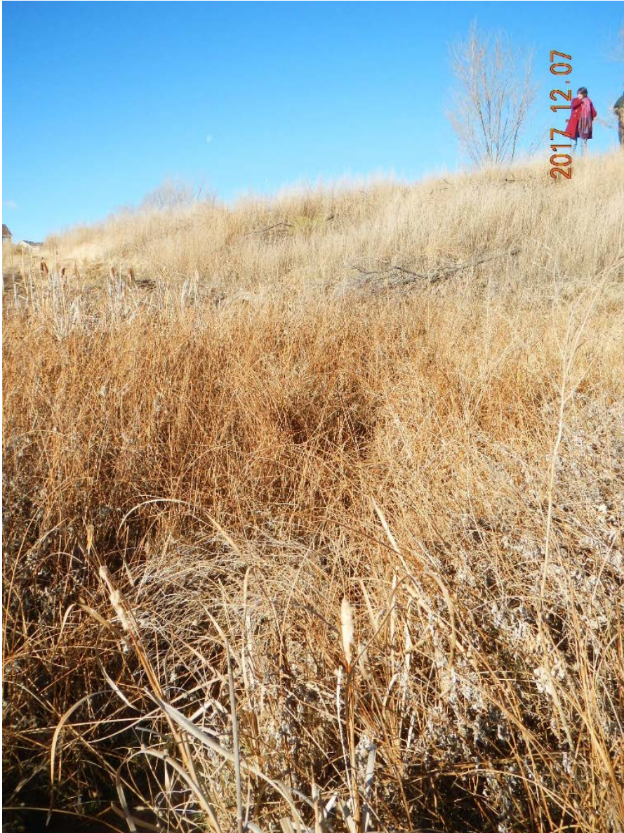
11_Downstream Slope, above old outlet
