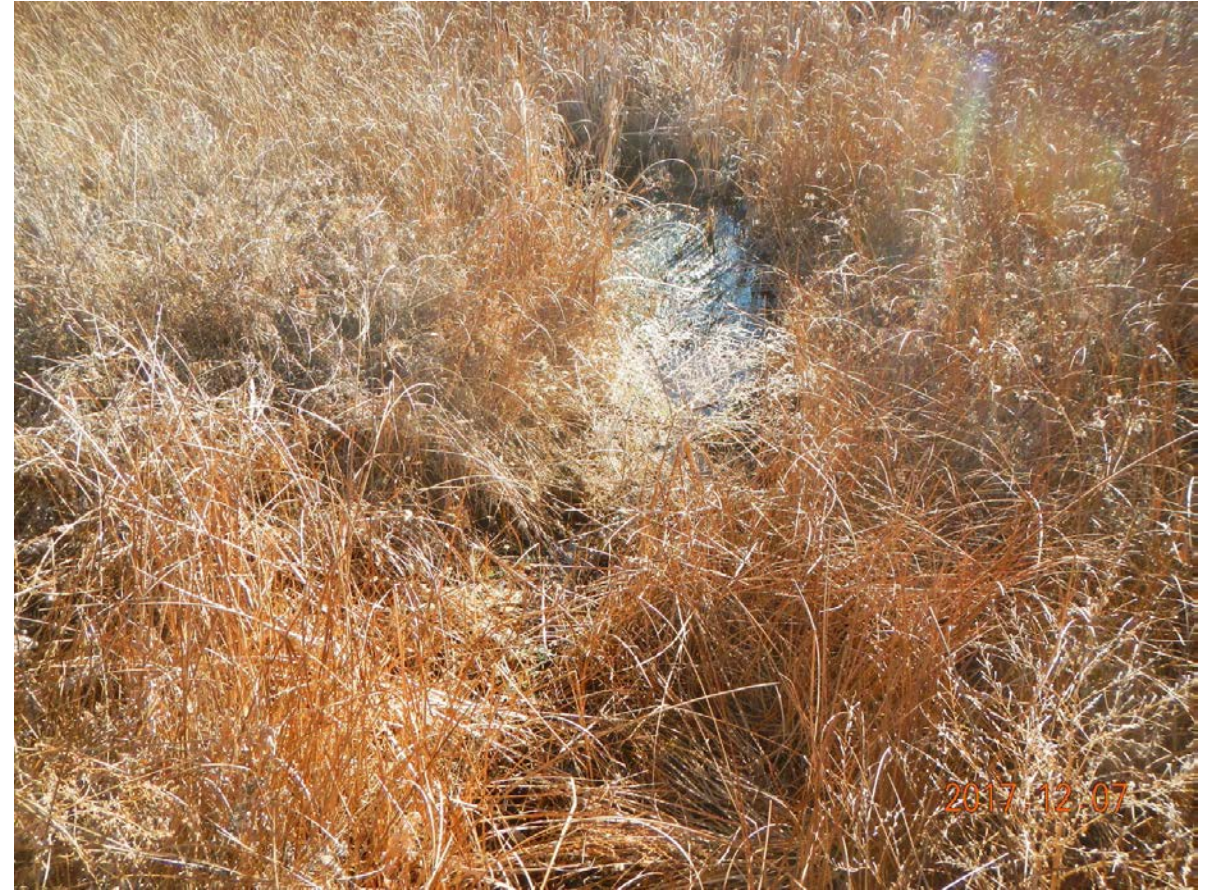
20_Seepage area left of old outlet
