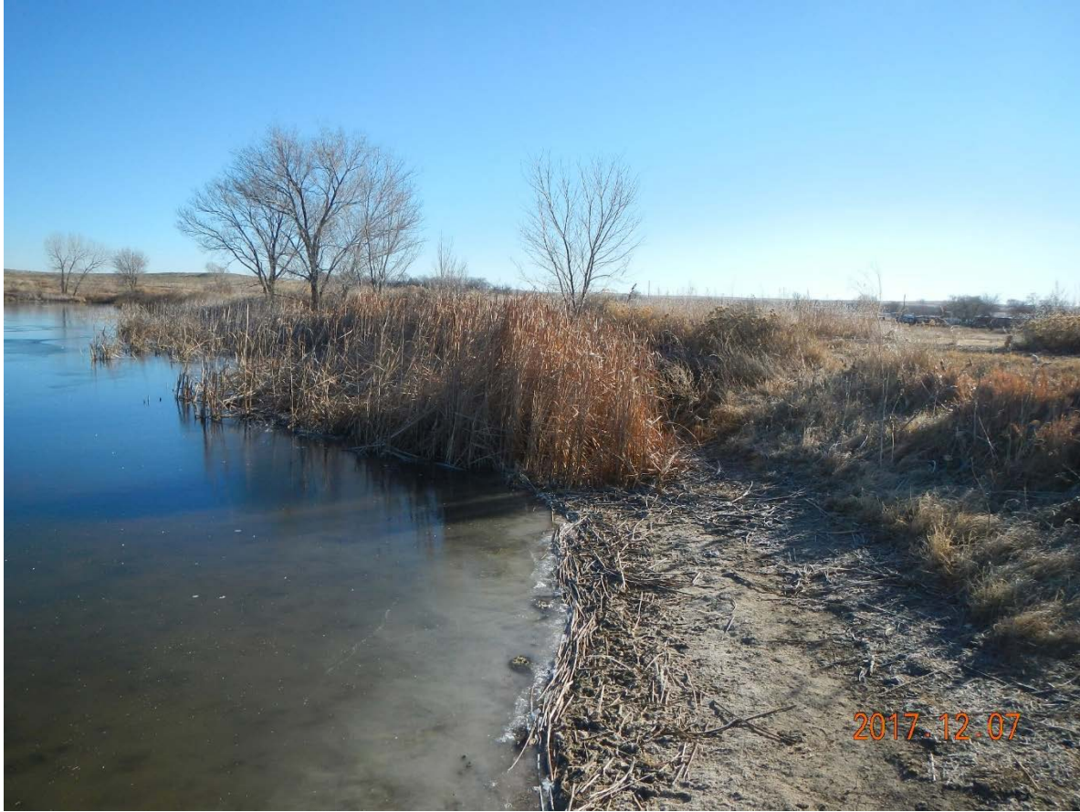
01_Upstream Slope, from right abutment
