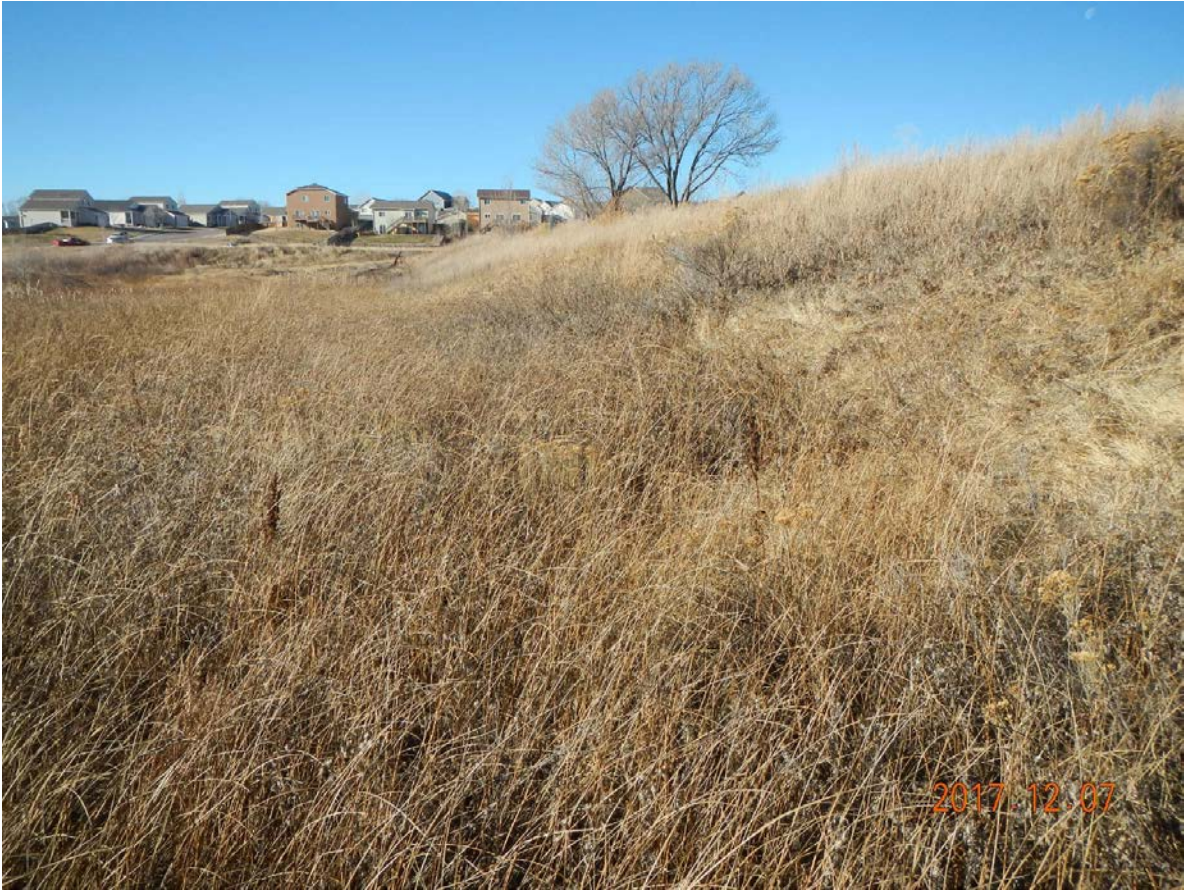
10_Downstream Slope, looking right at central portion
