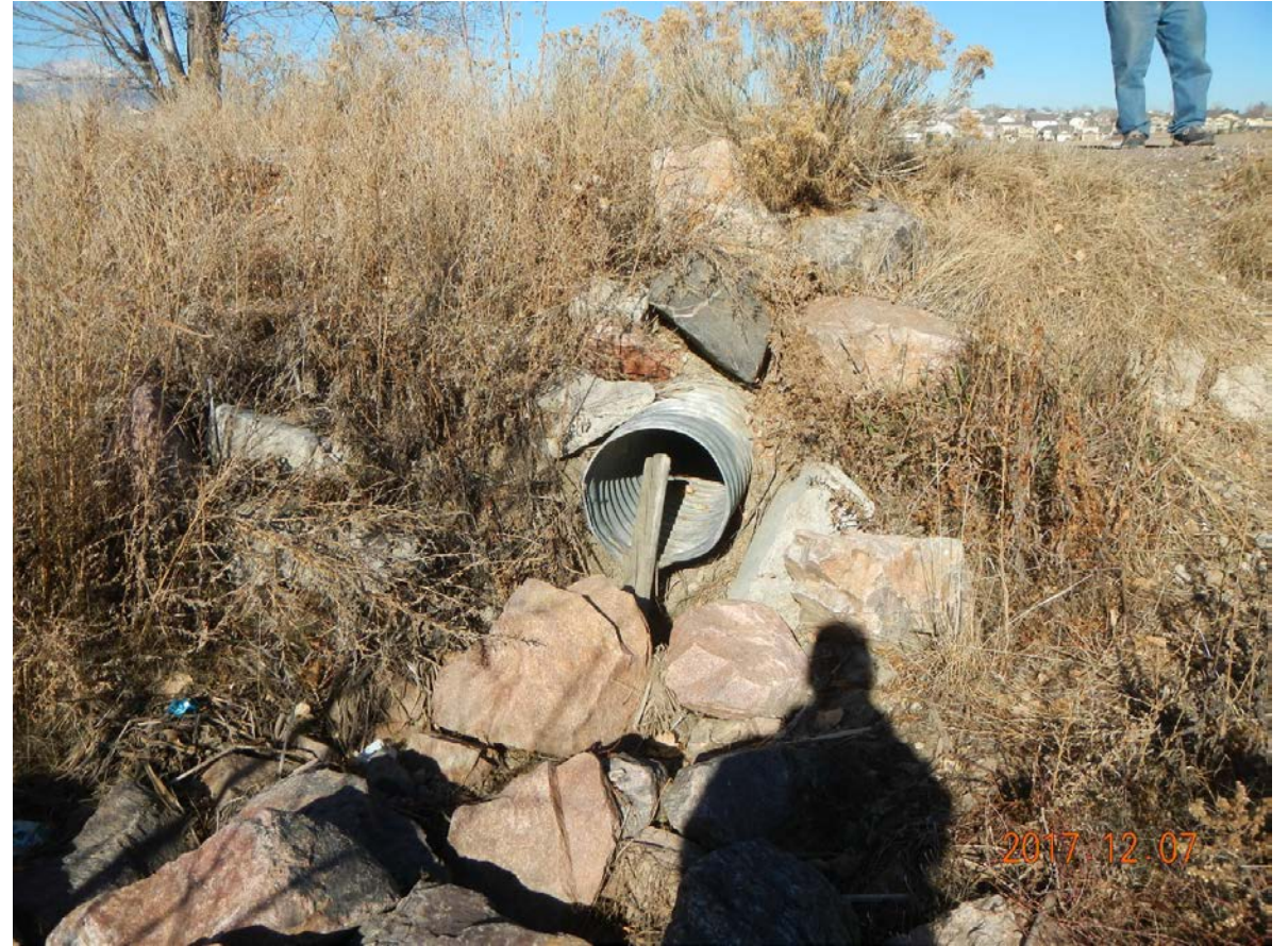
22_Pipe spillway on left end of dam
