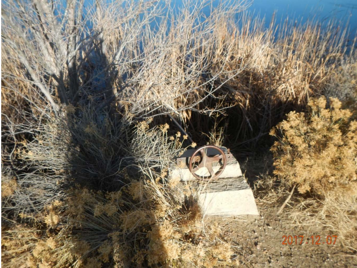
15_Outlet, old operator
