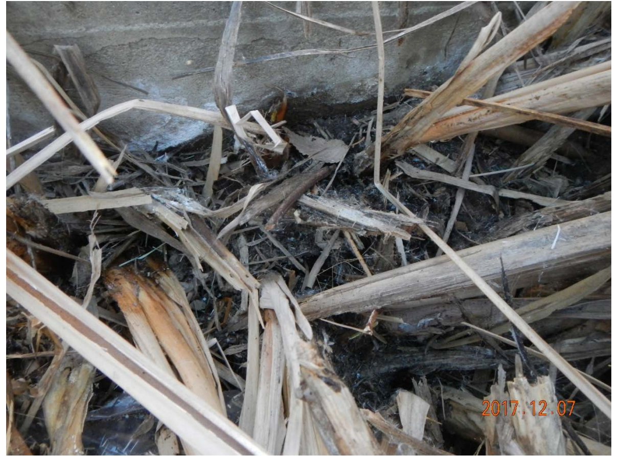
18_Outlet, old discharge point concrete
