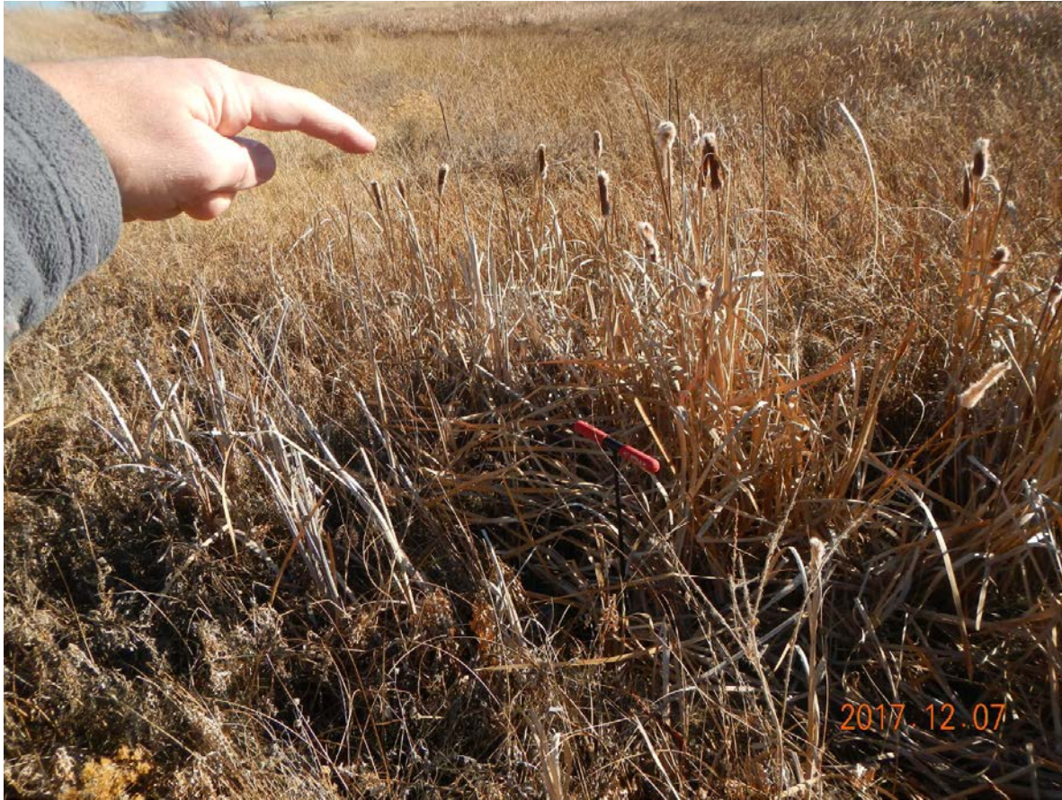
19_Seepage area left of outlet
