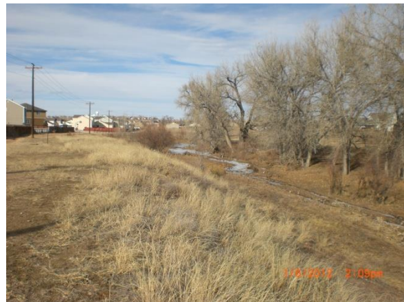
Typical grass lined channel
