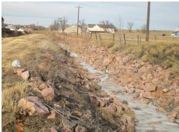
Typical rip-rap lined channel
